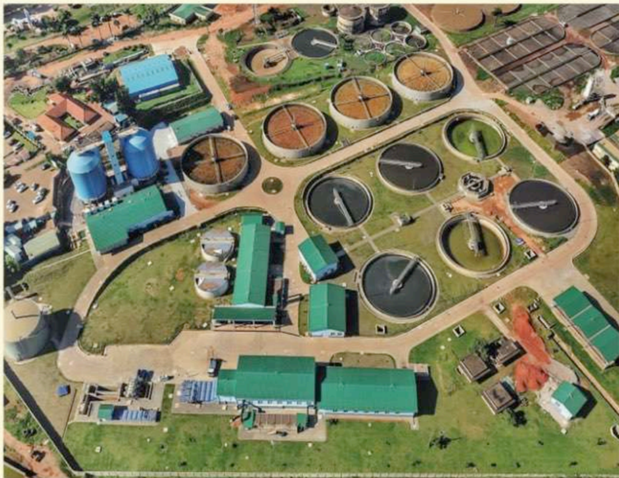
Construction works at Katosi water treatment plant
