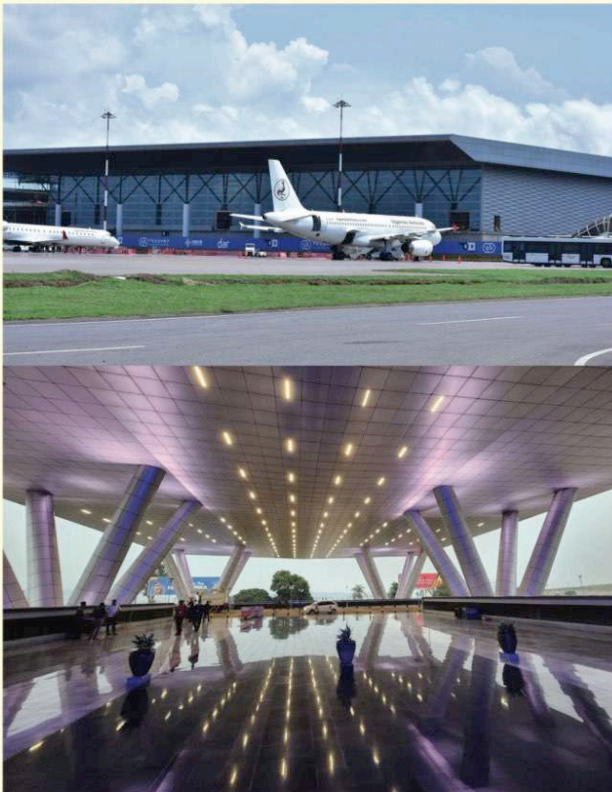
The newly rehabilitated Entebbe International Airport
