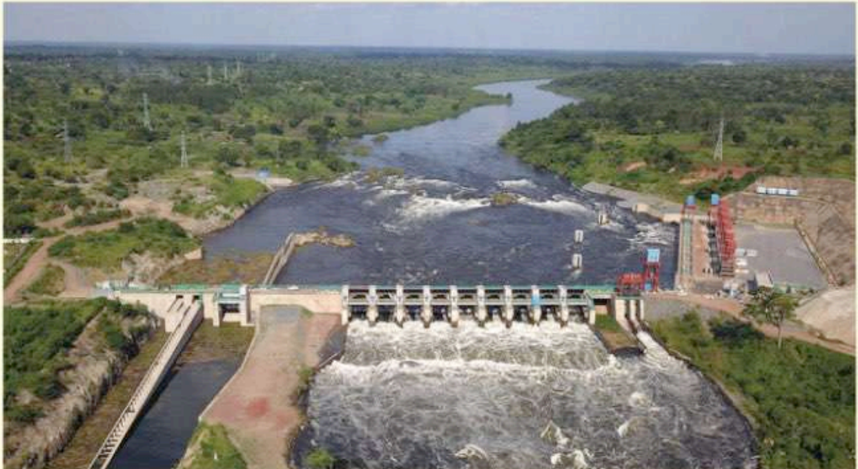
Karuma Power Generation Dam
