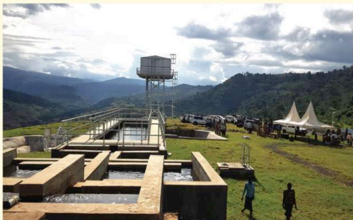
Bukwo Water Treatment Plant
