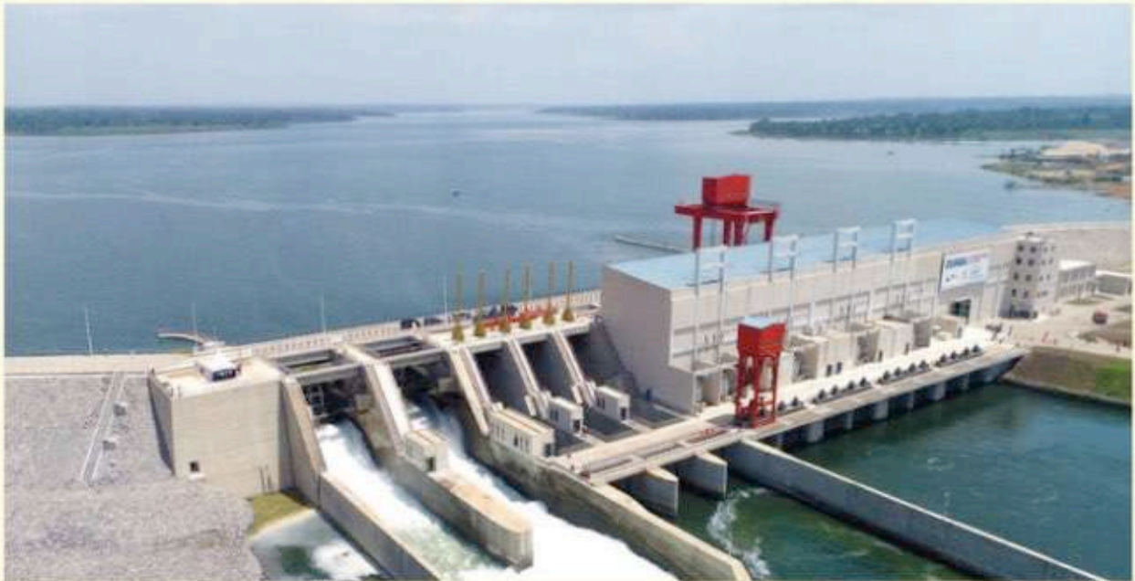
Isimba Power Generation Dam
