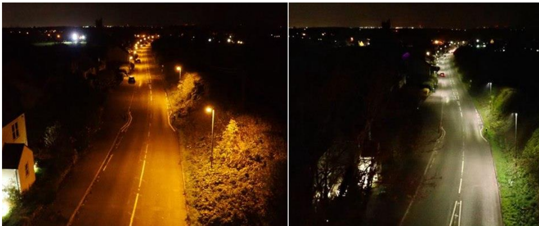
Figure 8: Street lighting with HPS Lamps Vs LED lamps
