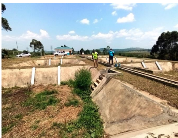
Plate 8: Effluent treatment facility in Buwama town
