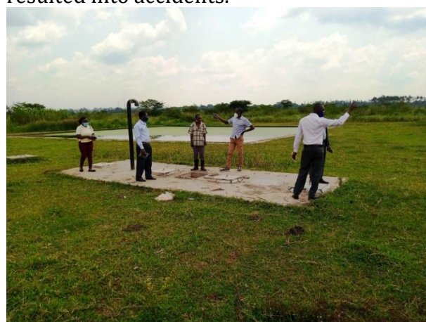
Plate 7: Effluent treatment facility in Kayunga
