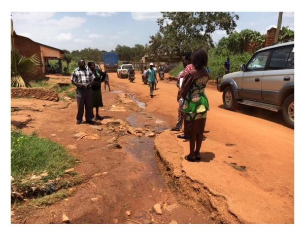
Lack of drainage system and road erosion in Kitgum
