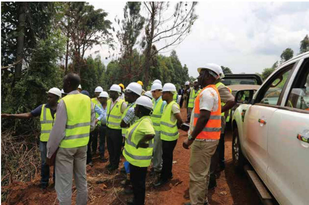
Across section of project officers inspecting the road works with emphasis on the forest reserves in Hoima district
