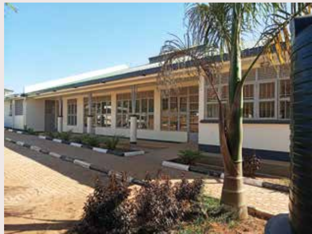
Multi-purpose Hall at the ISLM was constructed
