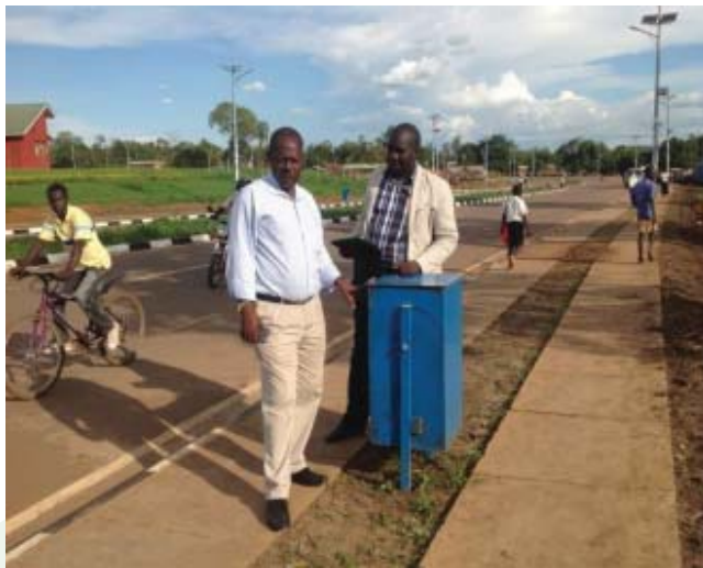
Walkways & dust bins on one of the USMID Roads
