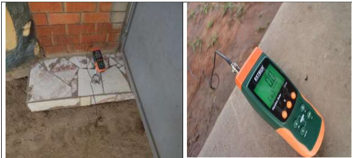
Figure 6: Deployment of the Vibrations Monitor
