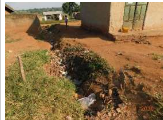
Waste collecting in the road drainage channel
