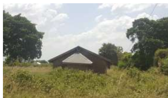
Figure 4-35: Buliisa Town Mosque along Kalolo road
