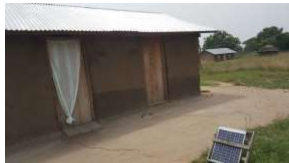
Figure 4-70: Iron roof house along Rif Valley road
