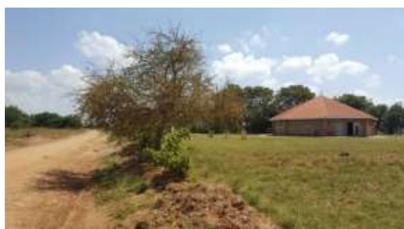
Figure 4-34: Buliisa Town catholic church along Galende road
