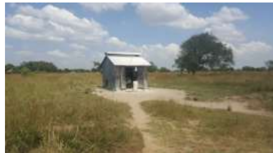
Figure 4-47: Grinding mill along Gongo road
