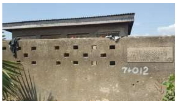
Figure 4-73: A VIP latrine in Butiaba market constructed by Biiso Subcounty
